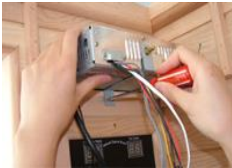
FIG-16.2 Fix the CD to the metal support
