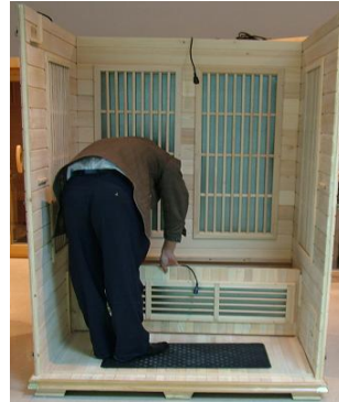
FIG-8 Assembling sitting board's support
