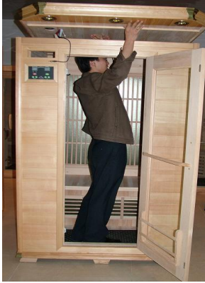
FIG-12 Setting the top board
