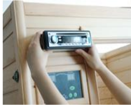
FIG-16.1 Fixing stereo w/ CD
