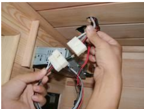
FIG-17 Link the CD connectors
